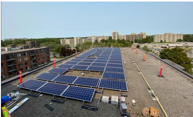
*Figure 11- 304 Oxford St., Solar Panel Installation*
