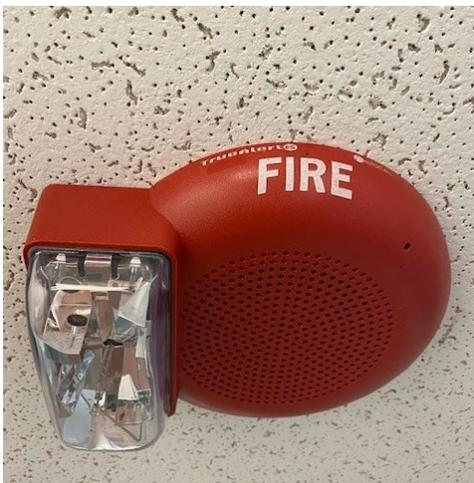
Figure 7- Tecumseh Ave., Fire Signaling Device
