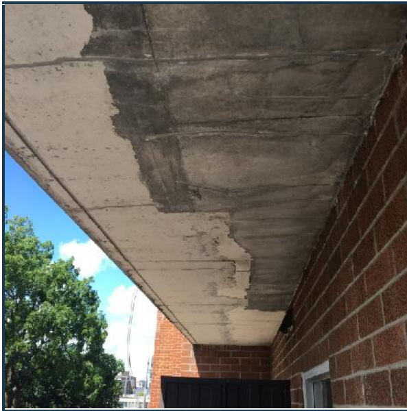
Photo 5: Evidence of uneven past repair.
