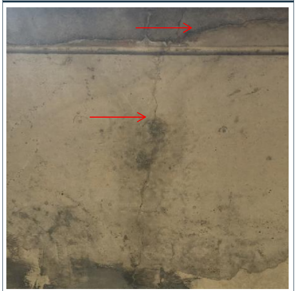
Photo 18: Soffit cracks.
