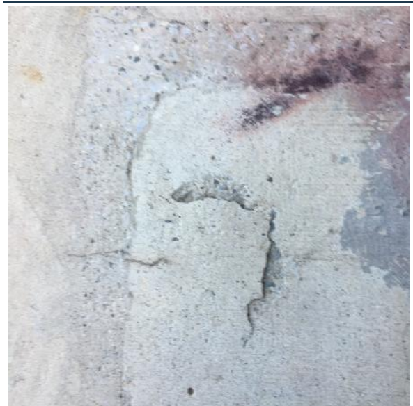
Photo 9: Front edge concrete delamination.
