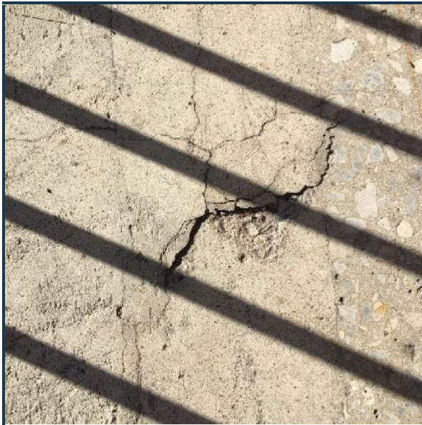
Photo 7: Topside delamination.
