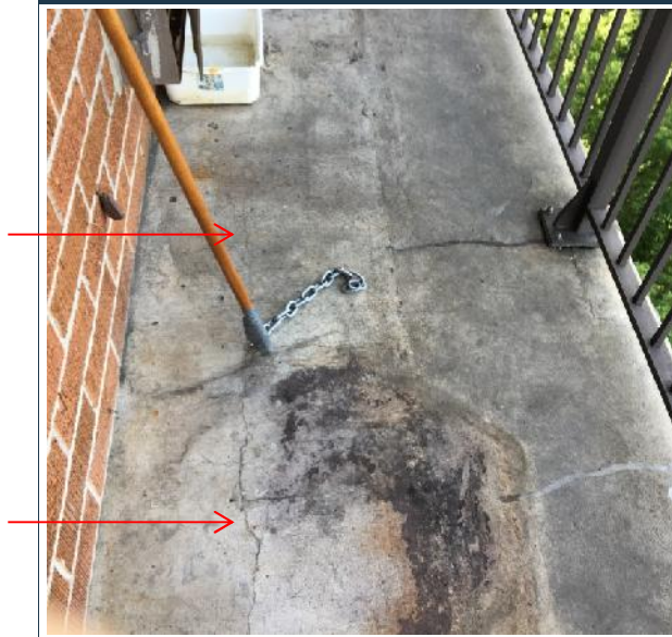
Photo 11: Top surface delamination along parallel bars.
