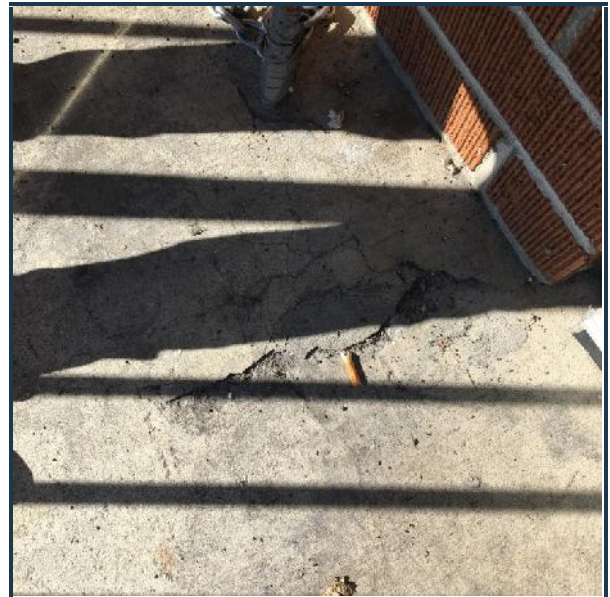
Photo 8: Topside delamination.
