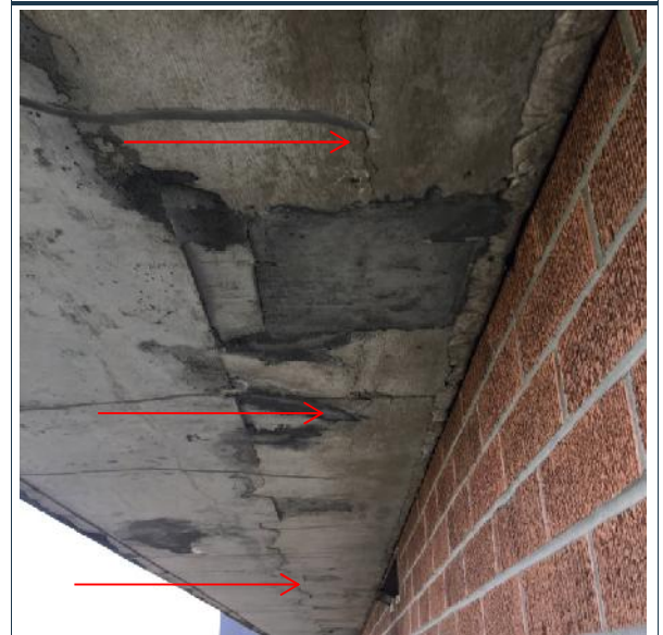
Photo 10: Crack running parallel to the exterior wall that requires a through slab repair
