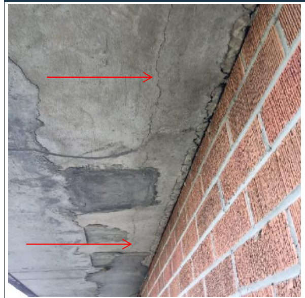
Photo 12: Soffit delamination and crack along parallel bars.
