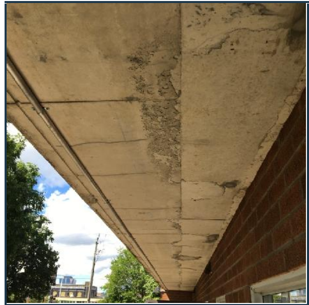
Photo 6: Evidence of chipping past repair.
