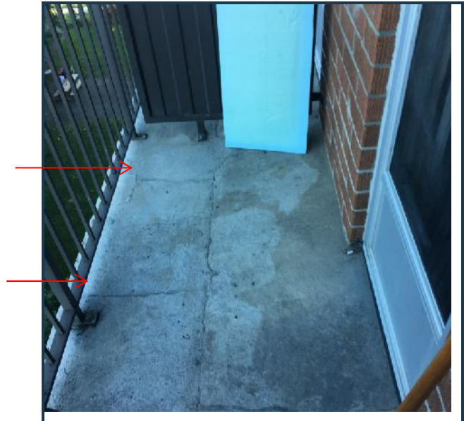
Photo 16: Topside cracks.
