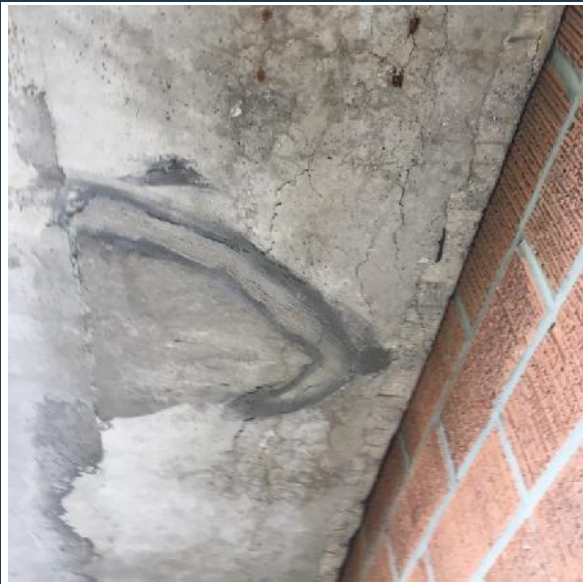
Photo 13: Soffit delamination and crack along parallel bars.
