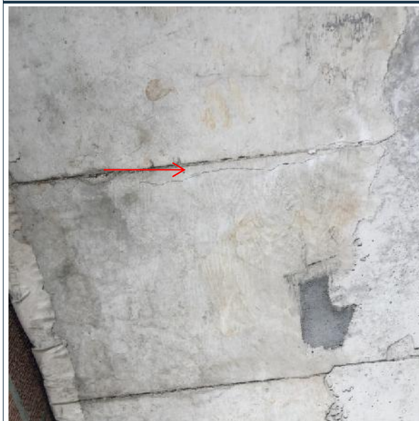
Photo 17: Soffit crack.
