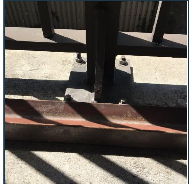
Photo 20: Guard baseplate anchored to concrete deck.
