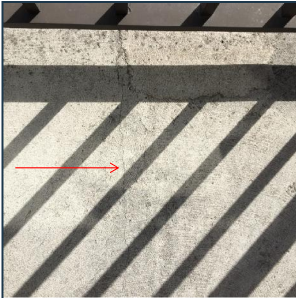
Photo 15: Topside crack.
