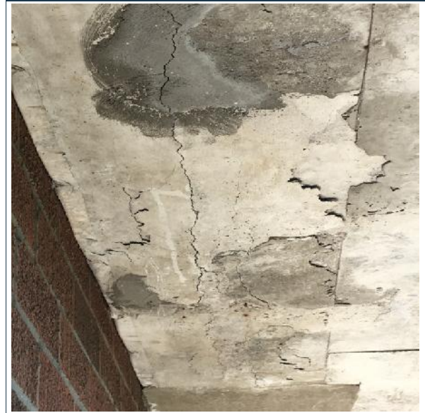
Photo 14: Soffit delamination and crack along parallel bars.
