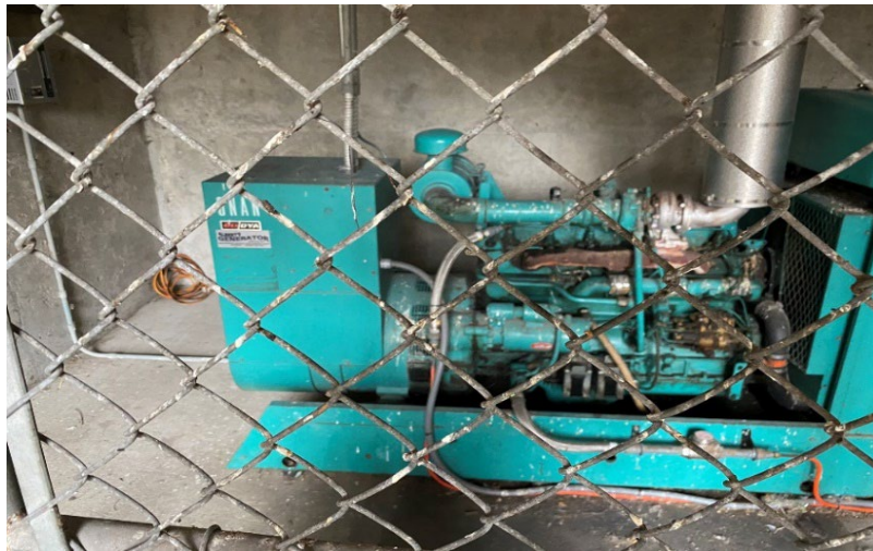
Figure 2 - New natural gas generator at Baseline
