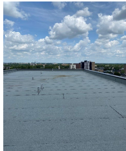
Figure 6 - New roof installed at Kent
