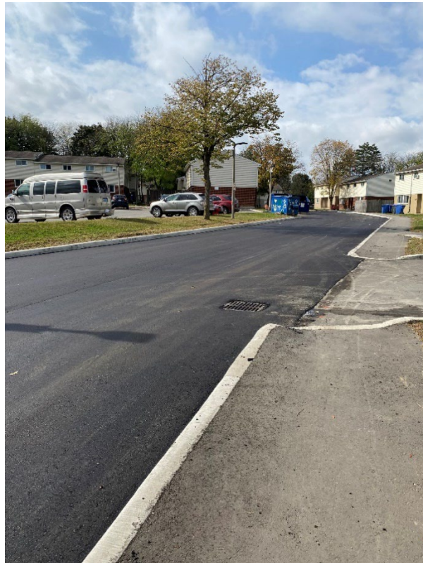
Figure 5 - Newly paved road and parking lot
