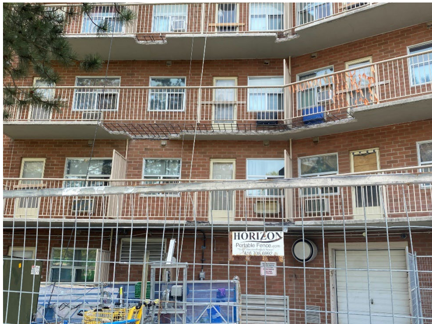
Figure 7 - Concrete balcony repairs underway at McNay
