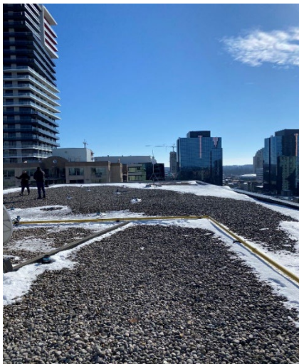
Figure 6 - Original roof surface at Kent St
